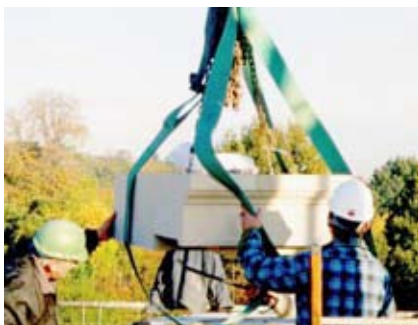
HALFEN stone anchors allowing easy installation of the coping stones.
