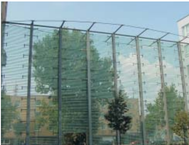
Noise protection wall, Oberlaa - Austria
