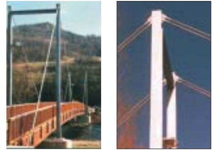
Pedestrian bridge, Schwarza - Germany
